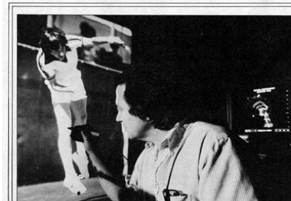
To analyze the body's efficiency, Ariel runs a film of the athlete through a computer, freezing each frame and measuring critical angles and lengths with a magnetic pen (left). The computer then creates a schematic printout (right)—in this case, of Jimmy Connors as he serves.
